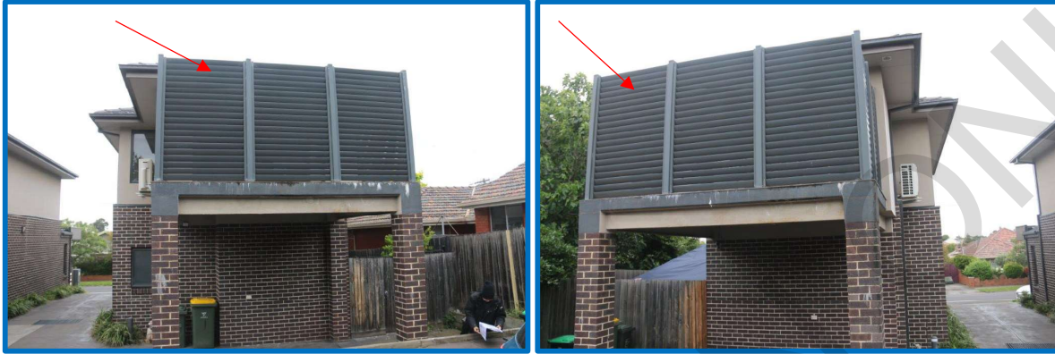
Figure 10&11: Louvred Metal Panels.
