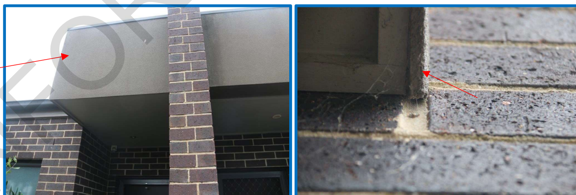
Figure 8&9: Cement sheet cladding
