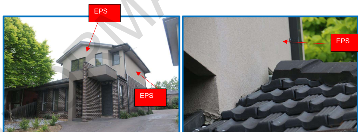
Figure 2&3: Townhouse 6 – Level 2 external walls constructed from EPS
