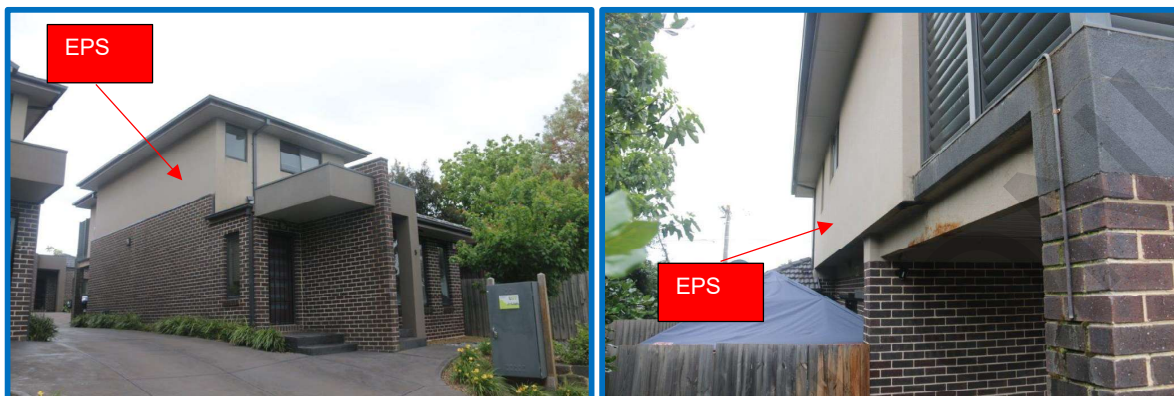
Figure 4&5: Unit 7 – Level 2 external walls constructed from EPS
