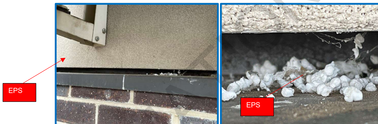
Figure 6&7: EPS Cladding
