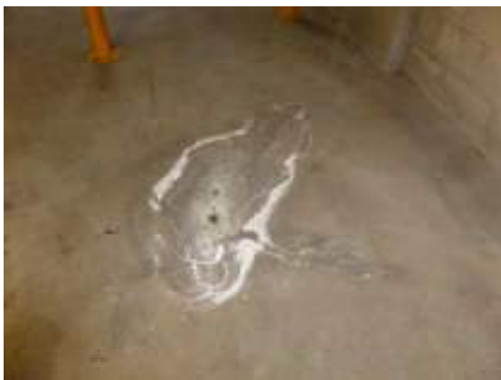
Photograph 8. Efflorescence deposits on the basement floor.
