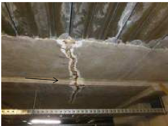
Photograph 7. Efflorescence extending across the ceiling and down concrete beams in the basement.
