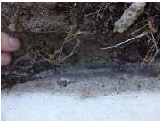
Photograph 3. Waterproof membrane not protected with a sheet membrane and did not extend 100mm above the ground level – which includes mulch.
