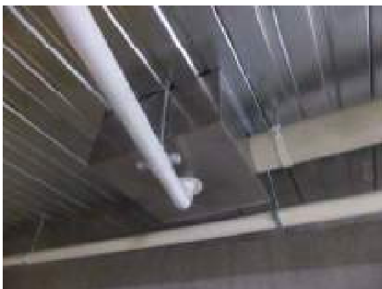
Photograph 11. Stainless steel tray which discharges via a PVC drain across the ceiling.
