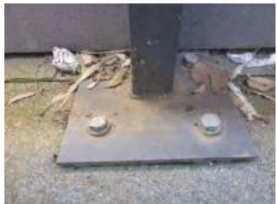
Photograph 18. Bolts through the membrane should be sealed to prevent water ingress.
