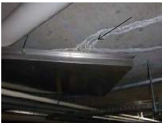
Photograph 5. Efflorescence stalactites formed on the basement ceiling indicating prolonged exposure to moisture.
