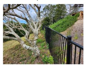
3. Area of pool fence is not closed off under the deck. This needs to be closed off with no gaps over 100mm.
