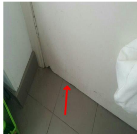
Moisture damage to laundry external access door. Repairs recommended to help prevent further deterioration.
