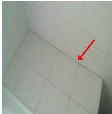
Recommend resealing bath hob at hob/ wall junction. A flexible sealant is recommended where differential movement takes place.
