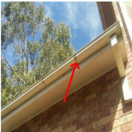
Corrosion to various gutter brackets. Rust treatment is recommended to help prevent further deterioration.
