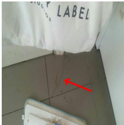
Cracked floor tile adjacent laundry external access door. Repairs aren't considered essential but would improve appearances.
