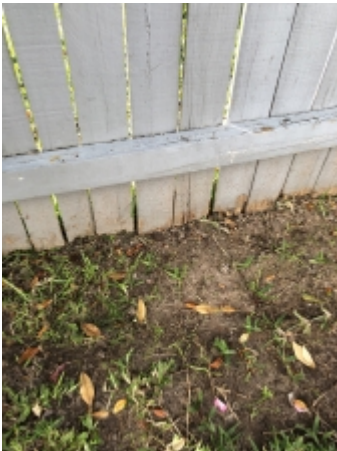
Timber in contact with damp soil
