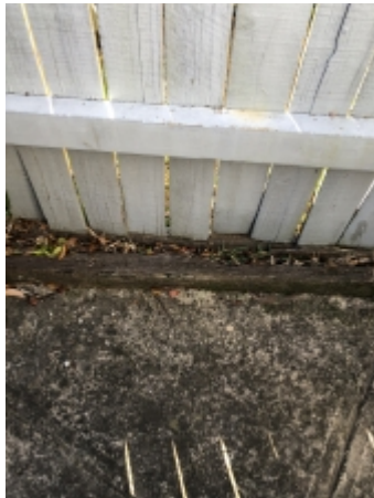
Timber in contact with damp soil
