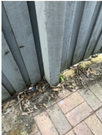
Timber in contact with damp soil
