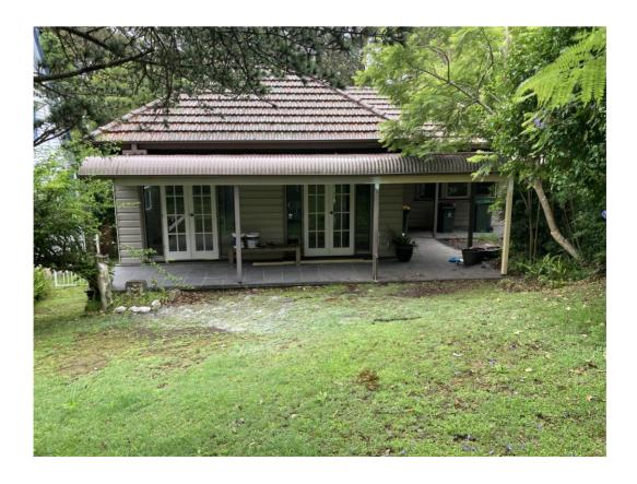
An inspection of the dwelling revealed it to be constructed from subfloor masonry walls and piers, and timber floor, wall and roof frames.
