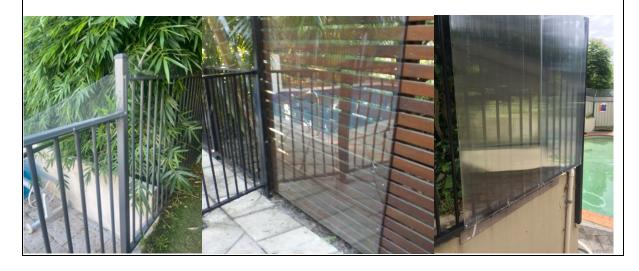
Vegetation was within the 900 mm Non-Climb Zone (NCZ) on the outside of the pool fence. The 900 mm NCZ is required to be kept clear so that children cannot use any object close to the fence to assist them to climb into the pool enclosure.
