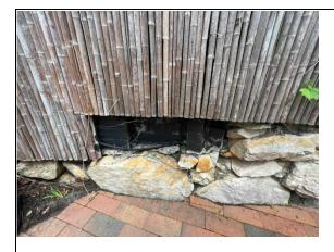
Below are some examples of ways to reduce gaps underneath a barrier.
