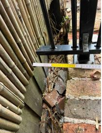
Below are some examples of ways to reduce gaps to less than 100mm.
