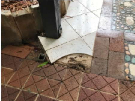
Showing example of cracked/missing floor tiles
