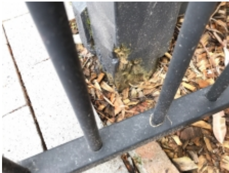
Showing example of wood rot
