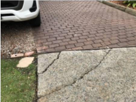
Showing example of movement cracking to driveway
