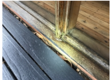
Showing example of wood rot
