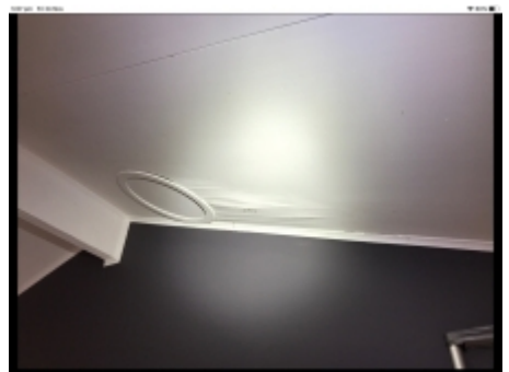
Showing dampness affected living room ceiling
