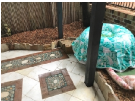
Showing example of timbers in direct ground contact
