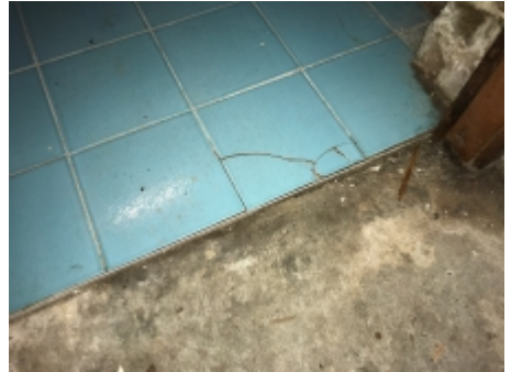
Showing example of cracked/missing floor tiles
