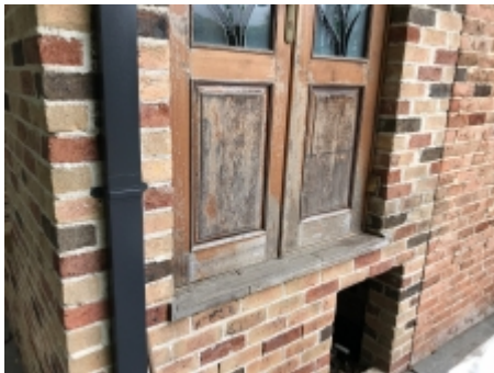
Showing example of weathered exterior timbers
