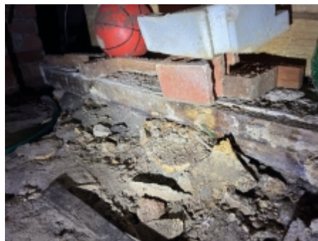
Showing example of timbers in direct ground contact to subfloor
