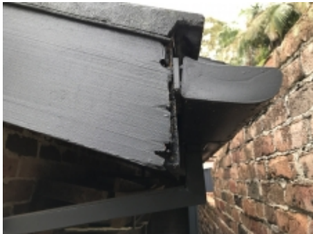
Showing example of wood rot
