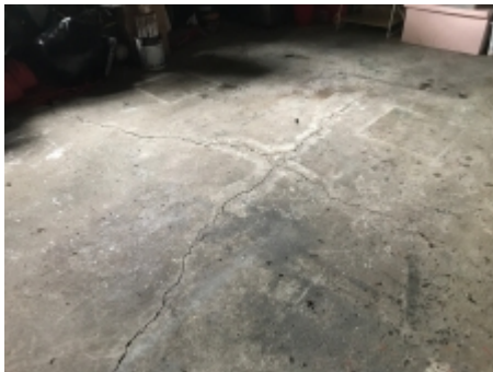
Showing example of movement cracking to garage floor slab
