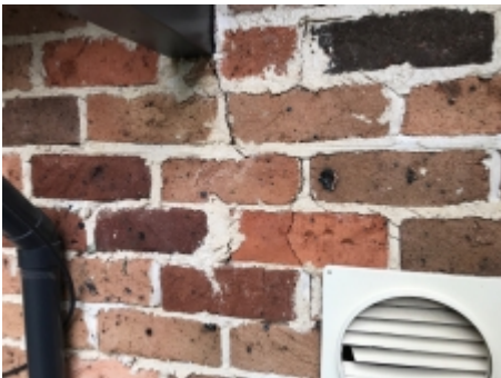
Showing example of settlement/movement cracking to external walls
