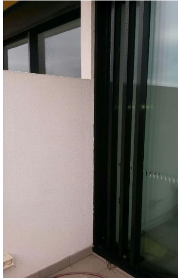
Figure 9 – Unit 39 sliding door
