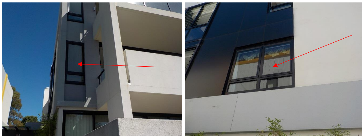
Figure 7 & 8 Windows to be replaced
