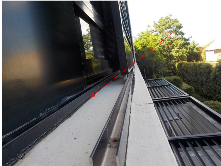
Figure 2 – Unit 25 & 33 FC cladding and window interface
