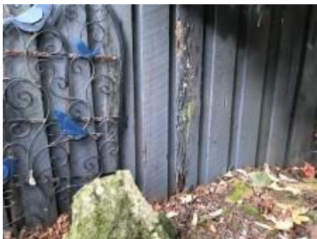
Wood rot to parts of the fences
