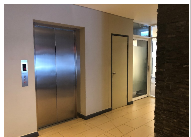
View of lift and commercial suite at ground level
