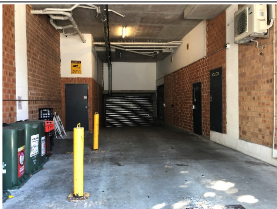
LOADING DOCK & PARKING ENTRY
