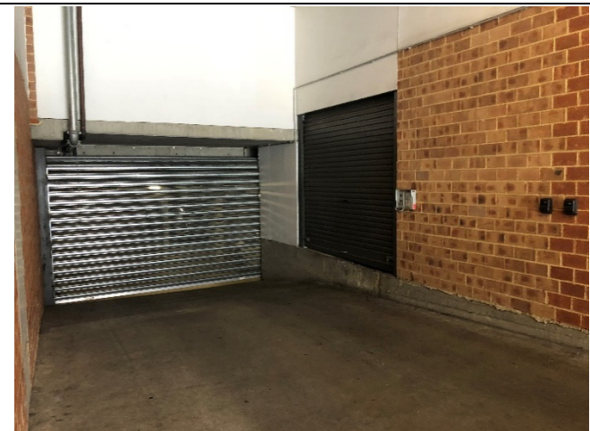
View of entrance to Basement and Loading Dock
