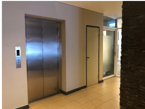
GROUND LEVEL FOYER
