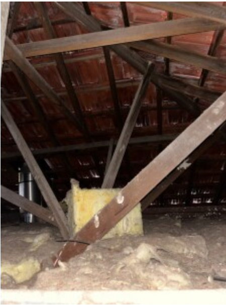
Roof void Insulated
