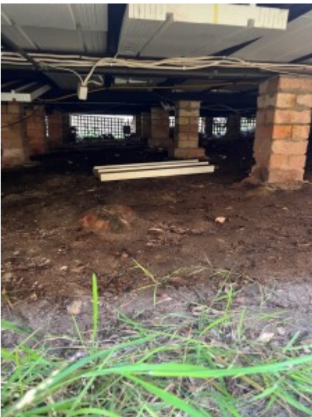
Sub floor Insulated
