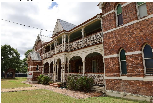
Face brickwork with rendered stringer courses.
