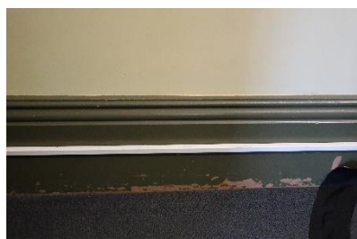
Timber skirtings. Note the later conduit is not significant.
