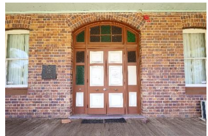
Original timber front door with coloured side and top lights
