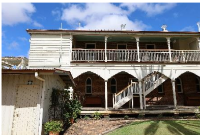
Open verandahs with timber balustrade and pointed arch valences.
