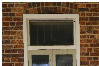
Louvre windows inserted in fanlights.
