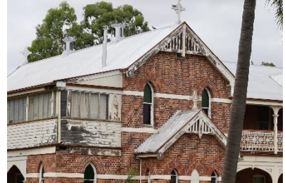
Red brickwork and corrugated metal roofing. Early timber weatherboard verandah infill. Chimneys, crosses and roof vents.
