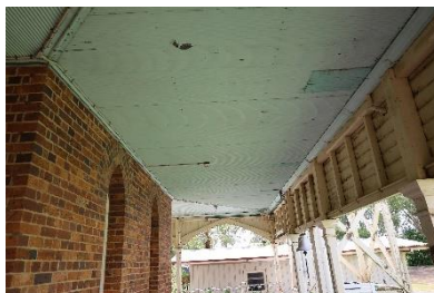
Verandah soffits including ripple iron and timber VJ boards.
