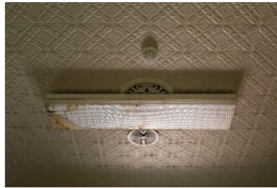
Modern light fittings and ceiling fans unsympathetically covering ceiling roses.
