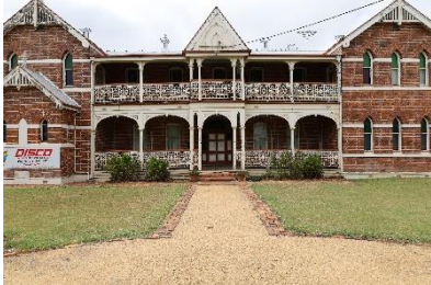
Front façade with central portico, timber verandah, cast iron balustrade and timber valance.
