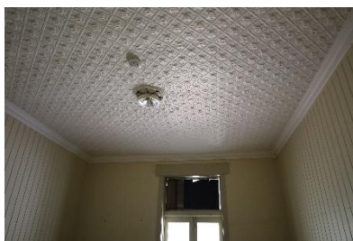
Pressed metal ceilings, ceiling roses and cornices.
