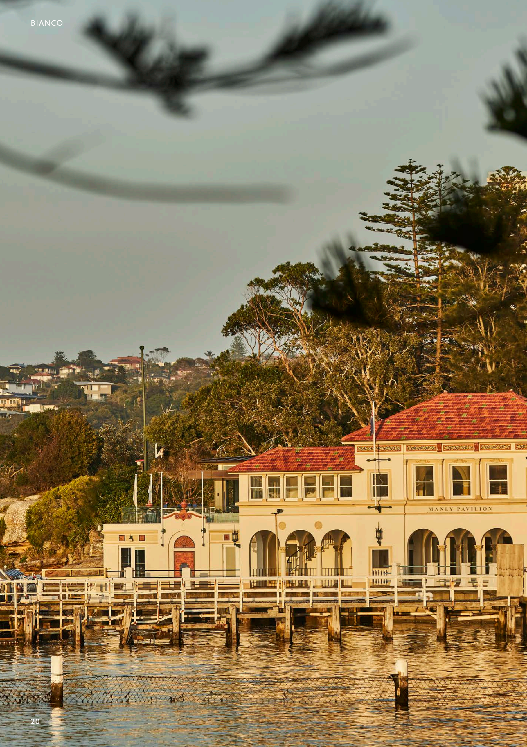
Manly Pavilion / Restaurant
