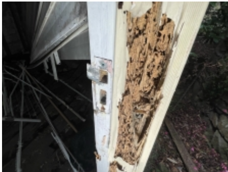
Termite Evidence / Damage
