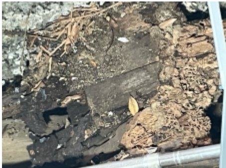
Termite Evidence / Damage
