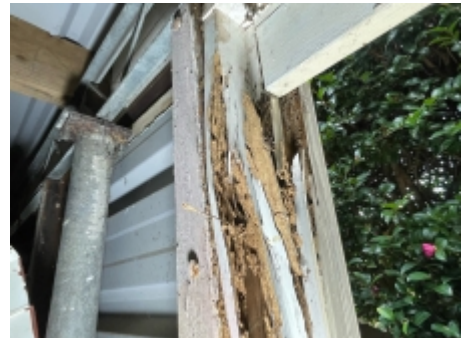
Termite Evidence / Damage
