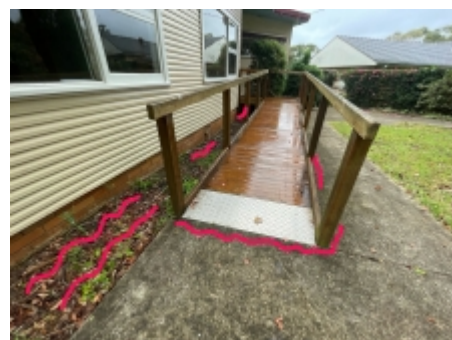
Poor Drainage / Bridging
