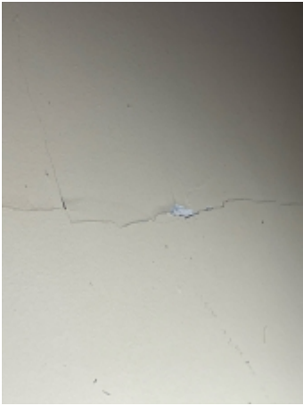
Hairline cracking - Plasterboard / generally
