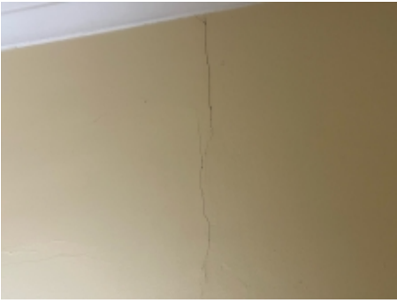
Hairline cracking - Plasterboard / generally
