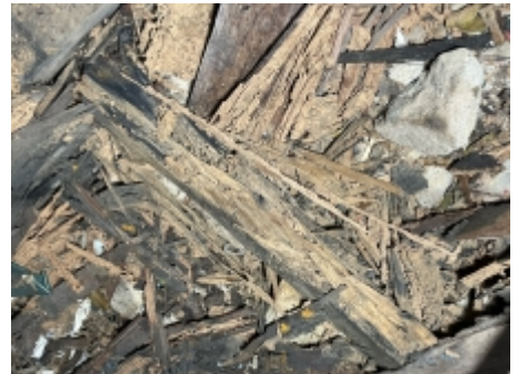
Termite Evidence / Damage
